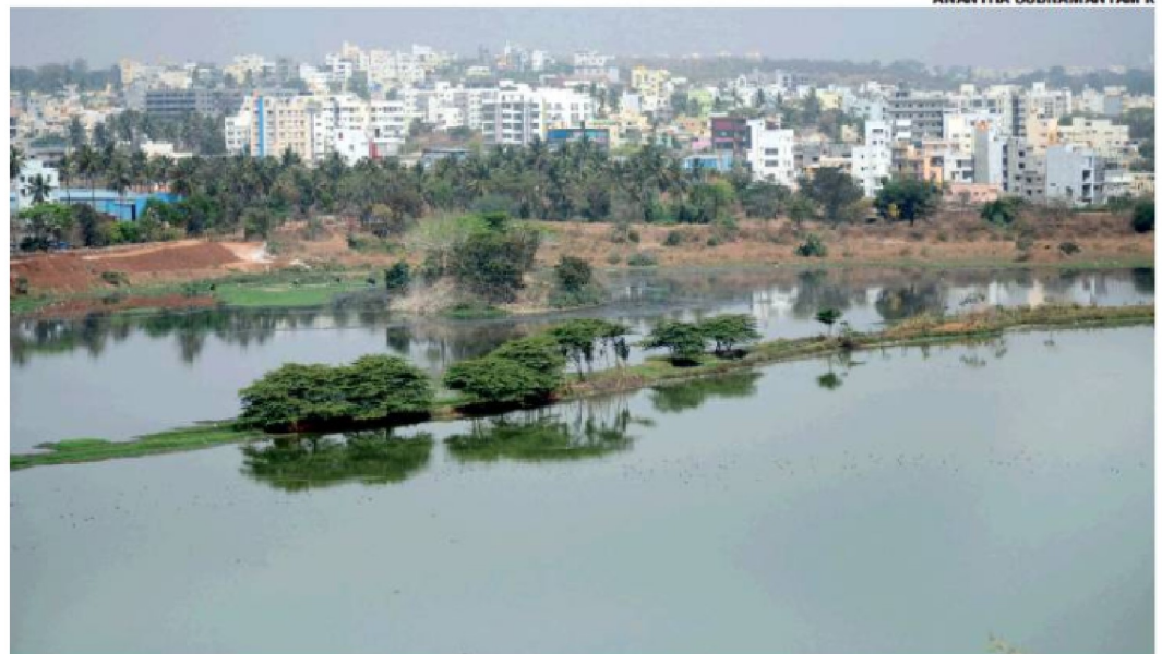
The retaining wall, he said, will be 3 to 4 metres in height and about 358 metres long
